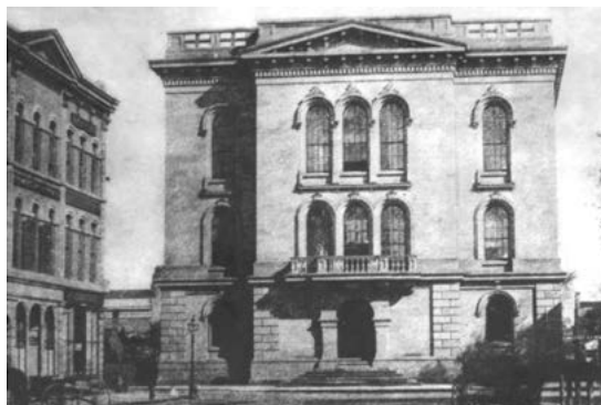
The Old County Courthouse on Public Square.
