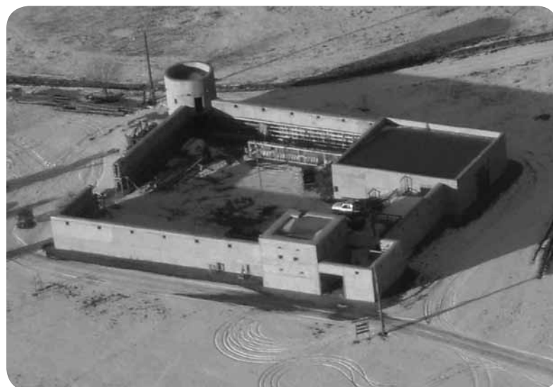
The fort as seen from the air during construction.
